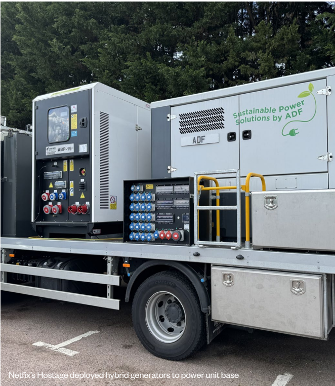
Netflix's Hostage deployed hybrid generators to power unit base
